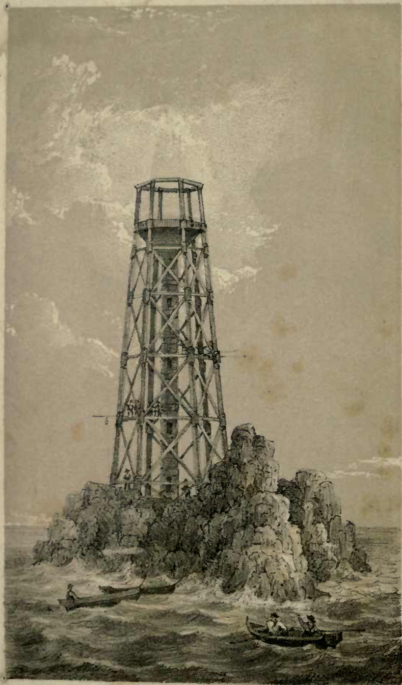
LIGHTHOUSE IN COURSE OF ERECTION ON THE BISHOP ROCK, as it appeared previous to its total destruction in the terrific storm on the night of the 5 th of February 1850
